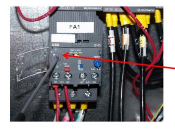
Reset the FA1 O/L relay setting using figure 1 chart below. Once set, close window.
